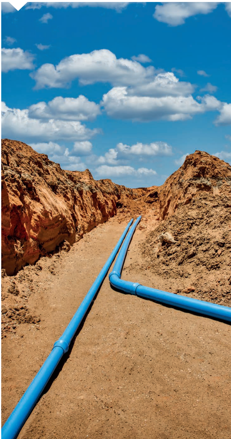
Installing new industrial PVC piping on a construction site in Botswana
