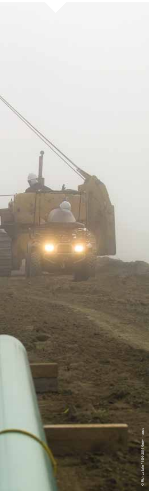
Laying a natural gas pipe at construction site in the fog.
